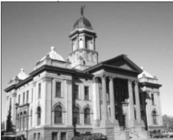
Above: The Cottonwood County Courthouse in Windom (1904) is an example of the Neo-Classic Revival style. It is listed on the National Register of Historic Places.
